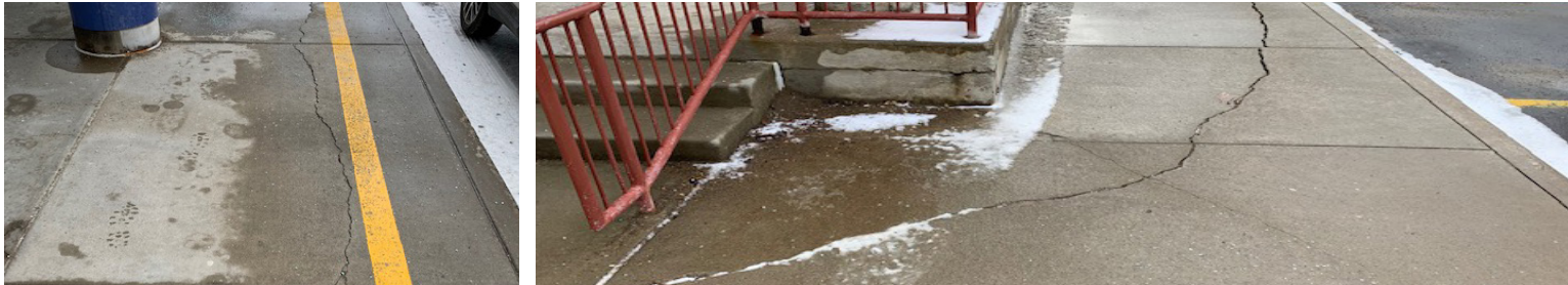
CRACKED SIDEWALK REPLACEMENT AT FRONT AND PLAYGROUND ENTRANCE
